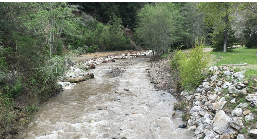
BEFORE: white rip-rap, failing bank
