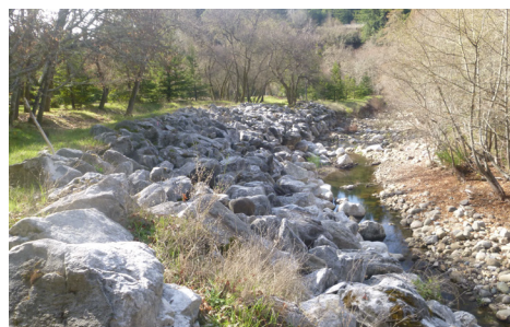
BEFORE: white rip-rap, failing bank
