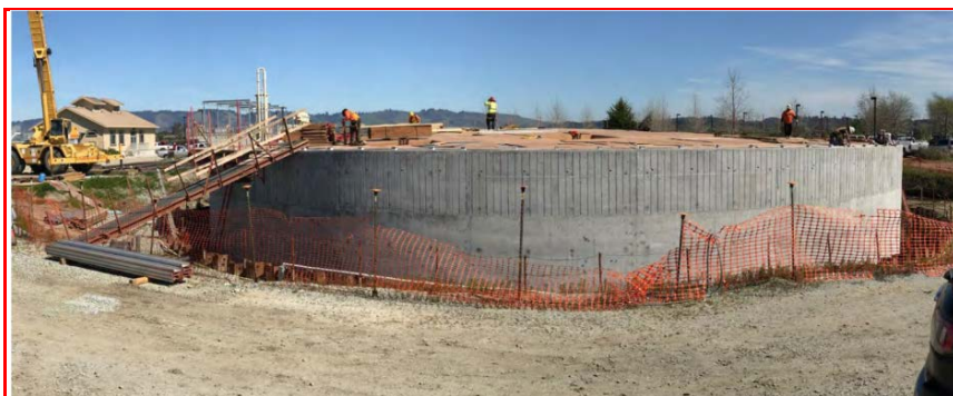
New 2017 Storage Tank at Recycled Water Facility
