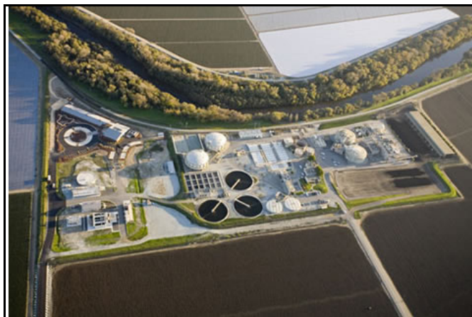
Watsonville Wastewater Treatment Plant and Recycled Water Facility
