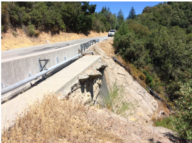
Hutchinson Road Viaduct, Summit
